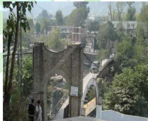
Fig:7.3 Suspension Bridge selected for retrofitting
