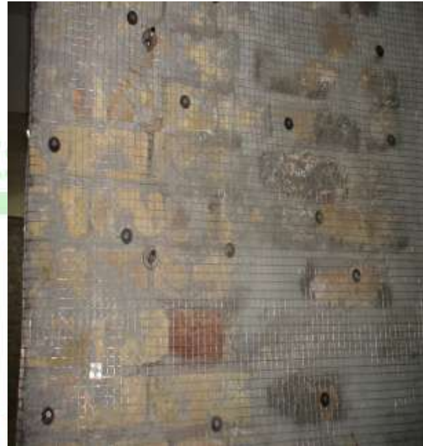
Fig:7.2 Retrofitted Wall of Jinnah Dental Hospital
